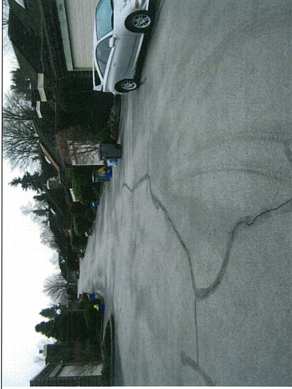
Photo 1: Photo dated March 4, 2009 looking north on Marchwood Place, showing pre-existing asphalt cracks.
